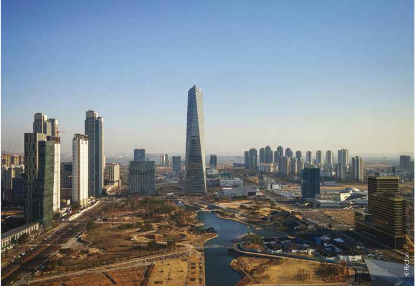
The headquarters of the Green Climate Fund are situated in the Songdo International Business District, South Korea
